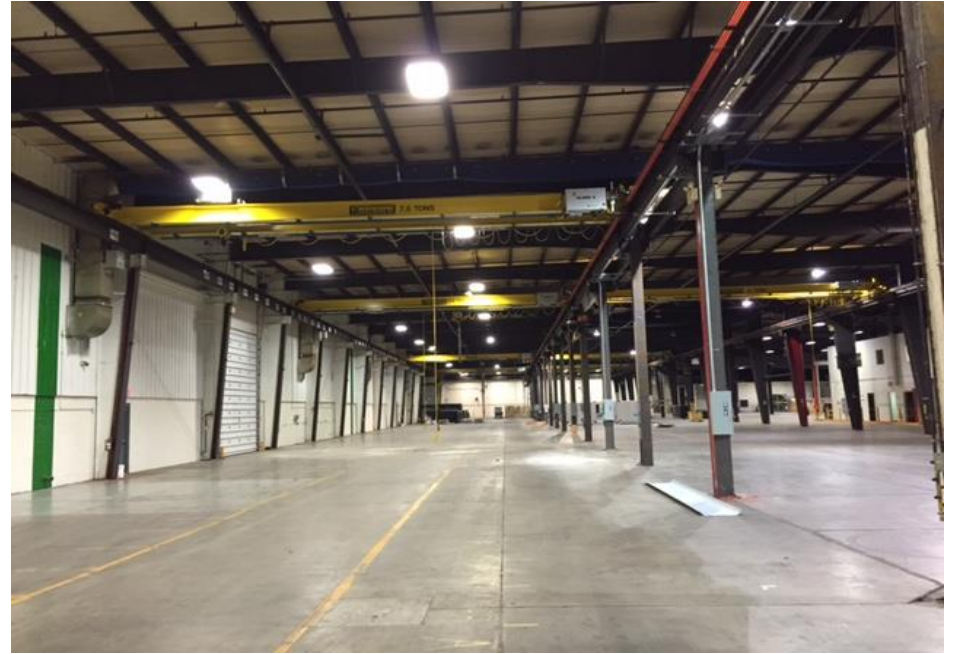
Typical 50' Crane Bay
